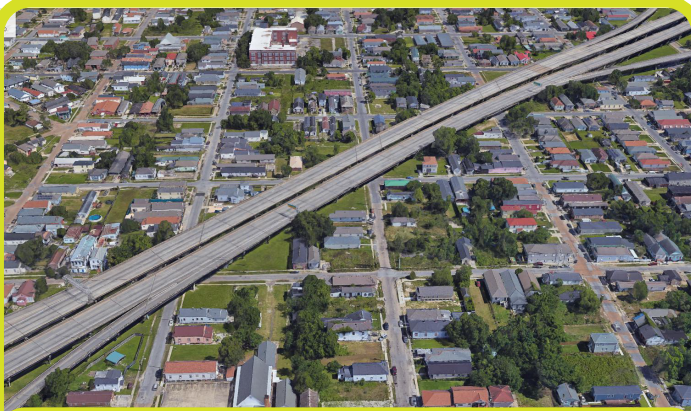
a Interstate-10 Detention Basins
